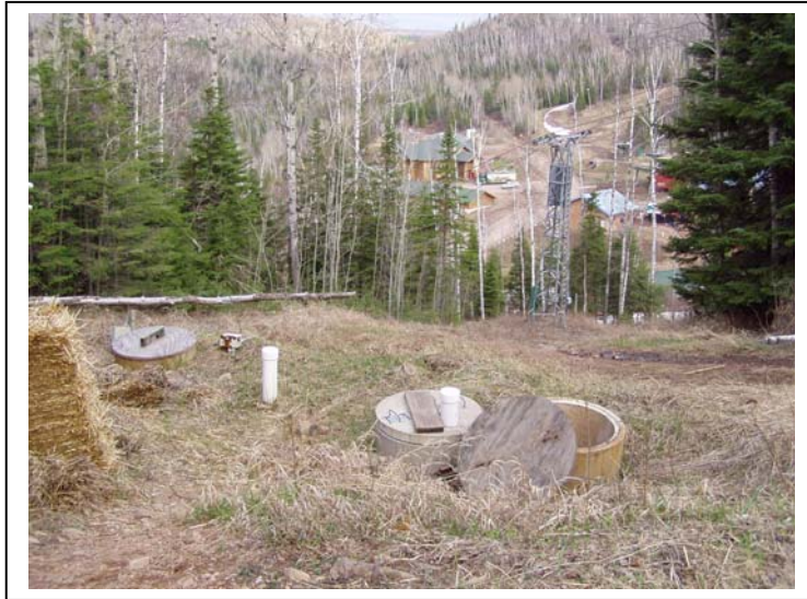
Figure 1: Settling tank on top of hill for the drip irrigation system.
